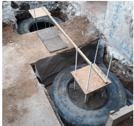
Figure 8: Diagram of Small building foundation using tires ( Critical Concrete 2019 )
