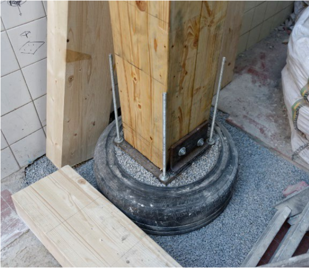
Figure 7: Tire House Foundation Support ( Critical Concrete 2019 )
