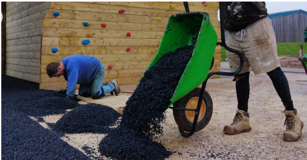
Figure 9: Installation of rubber and resin compound for playground flooring (Liberty Floor Solutions 2024).
