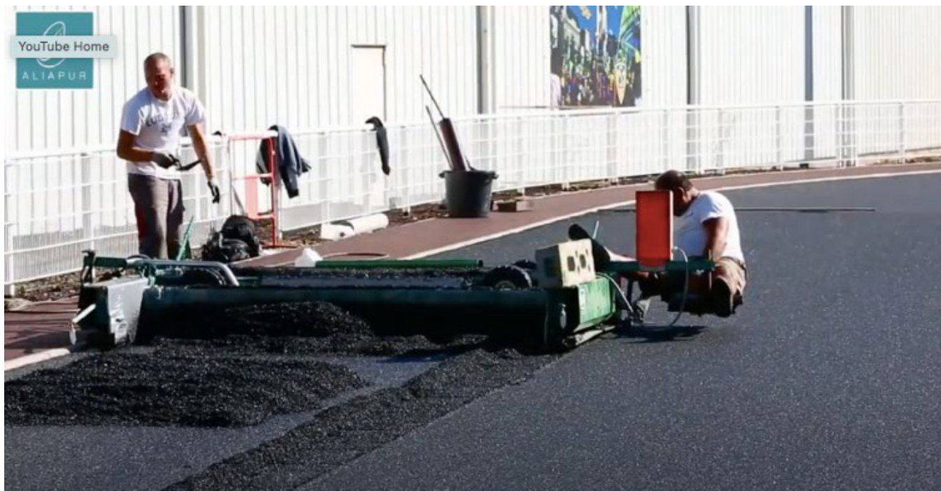
Figure 11: Athletic track constructed from Tires ( Communication Aliapur 2013 )
