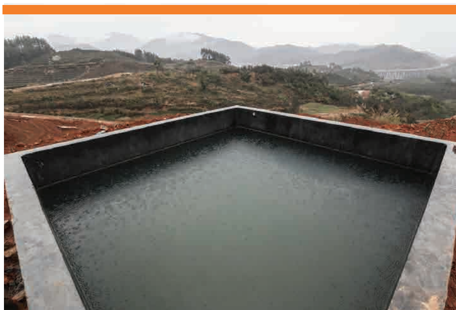
Rural innovation. In one of ADB's rural projects, mountain rainwater stored in a pool and used for irrigation or drip irrigation of tea trees during drought (photo by Lu Guang/ADB).
