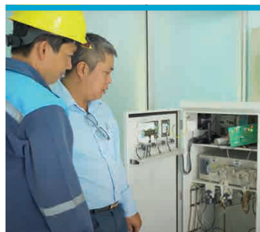
Real-Time Monitoring. A biosensor unit designed by EnvironSens, a Singapore-based startup, installed at SAWACO’s pumping stations in Ho Chi Minh City for river water toxicity monitoring (photo by Imagine H2O).
