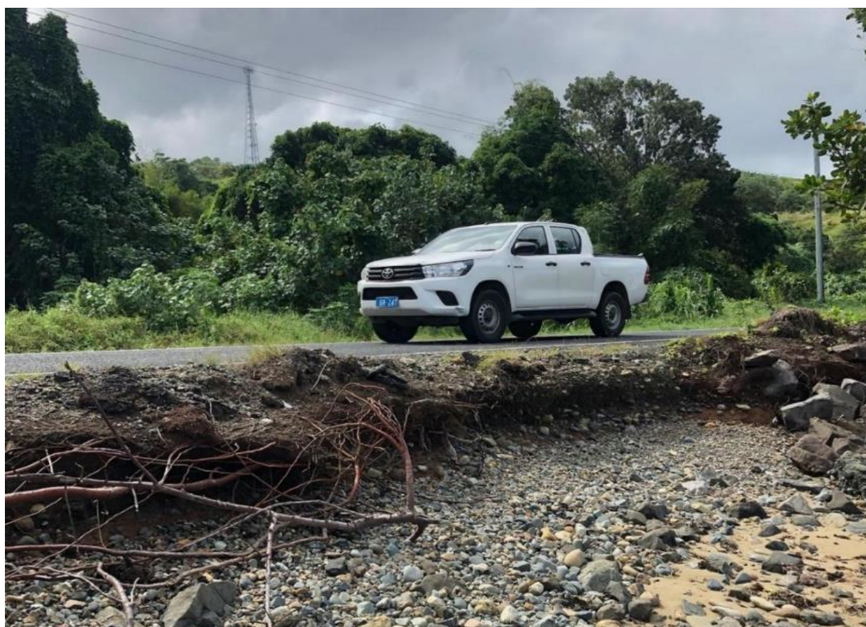
Figure 5. Erosion threatening transportation corridor near Galoa (May 2023)
