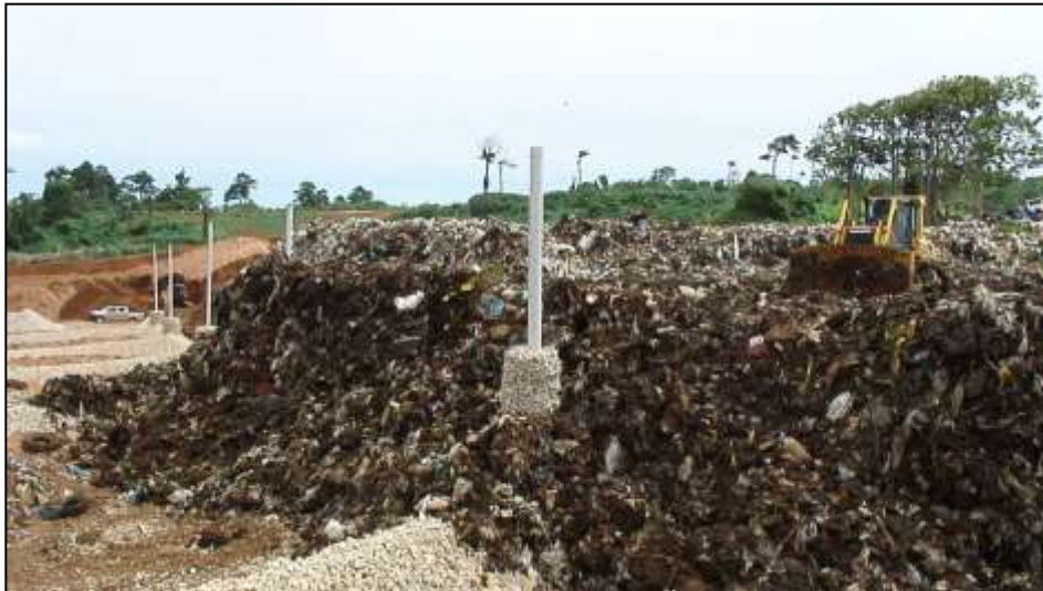
Backfilling Waste on the pipes
