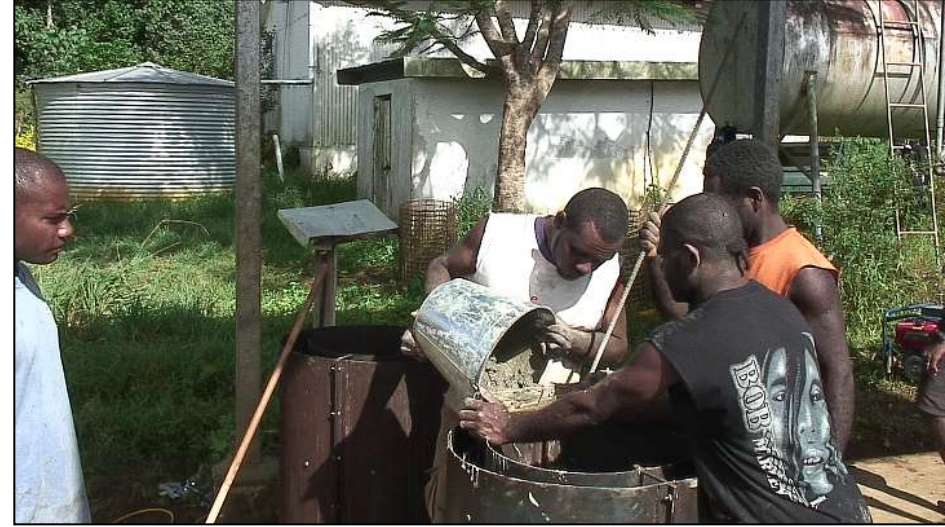
Casting Concrete
