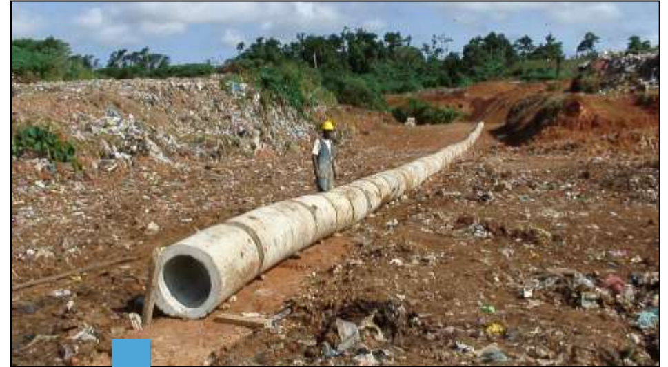
Placing Leachate Pipes
