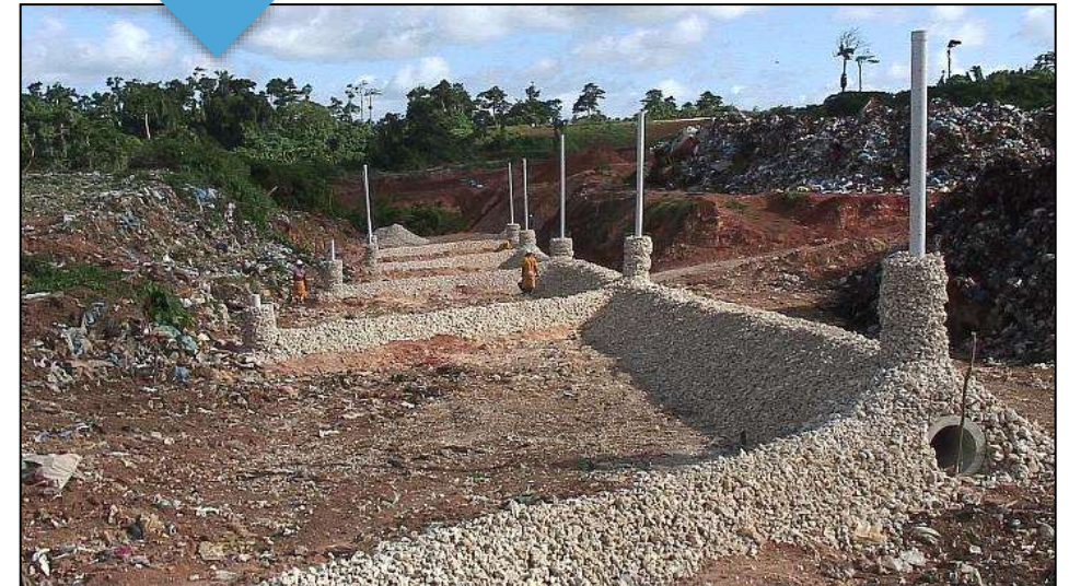
Building the Pipes Network with leachate/gas-vent Pipes
