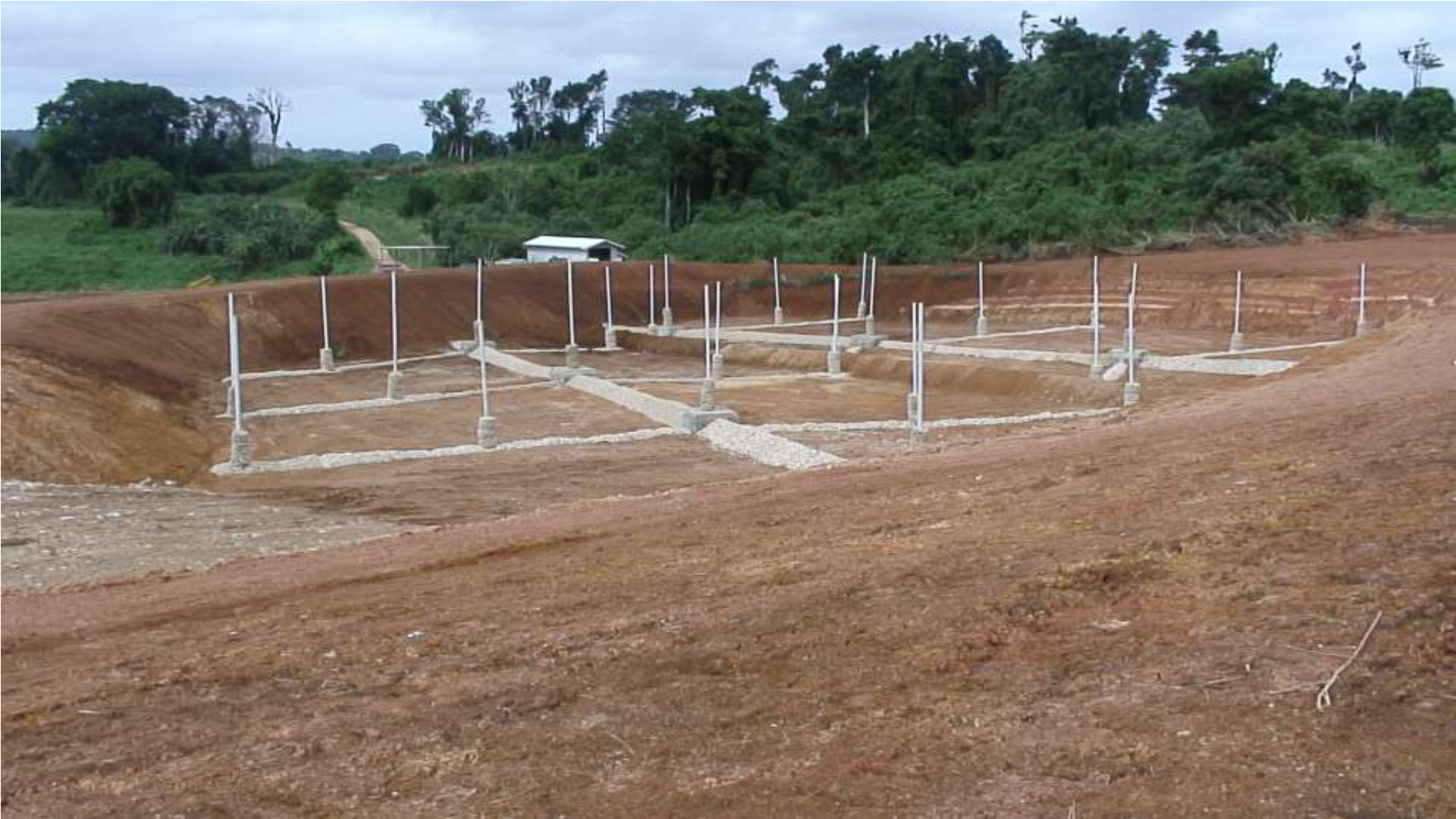
Built up Leachate Collection Network Pipe line
