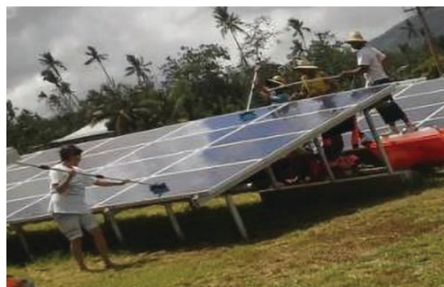
Figure 109: Erecting solar panels
