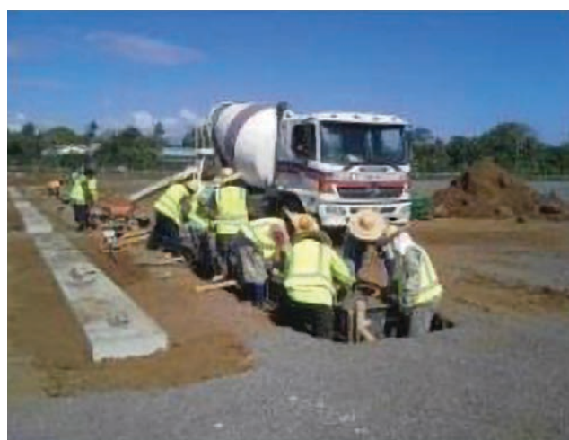
Figure 108: Footing prepares at the Racecourse Renewable Project.
