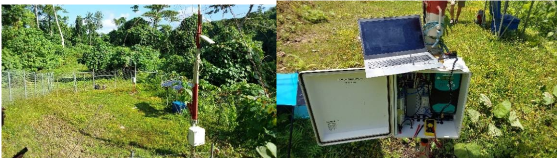
Figure A-3: Left image: Sarakata site enclosure. Right image: Logger/Sensor enclosure & testing.
