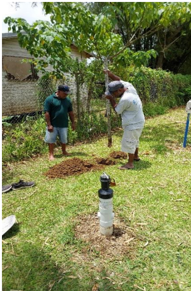
Figure A-1: Installing post – Sarakata School.
