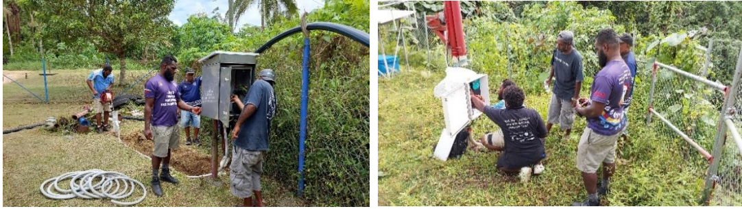
Figure A-2: Left image: Sarakata School install. Right image: Site commissioning..
