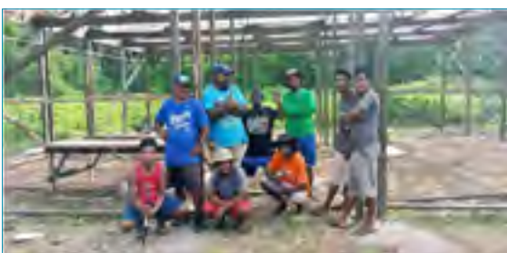
Completed greenhouse, Jaluit Atoll, Marshall Islands
