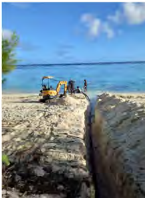
Installing the saltwater intake
