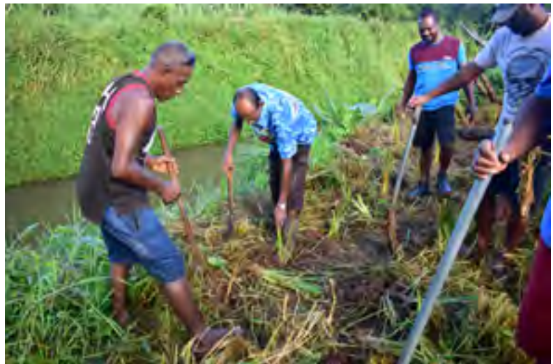
Planting vetiver grass to stabilise riverbank erosion in the Soasoa watershed, Fiji
