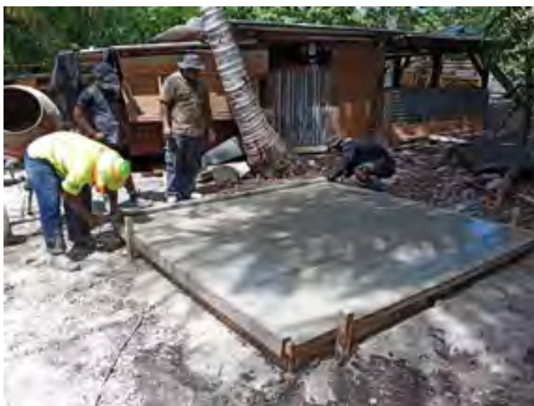
Installation in progress of tank base at one household, Nauru
