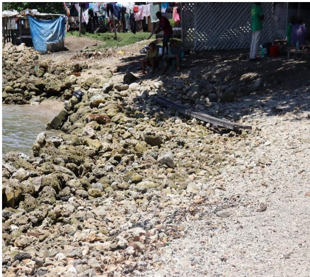
Fig.4.0 After Clean-up (West Side- -Bulky waste Removed)
