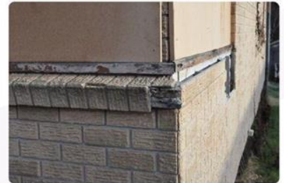
Imitation brick cladding
