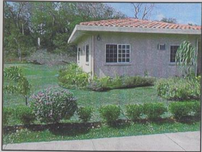
Figure 3.8 Rooftop runoff is directed to a landscaped area around this house in Saipan
