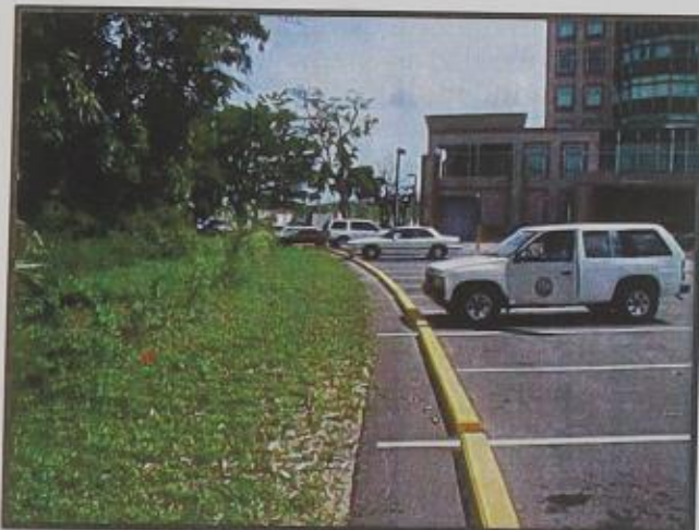
Figure 3.6 Use of a Grassed Filter Strip
