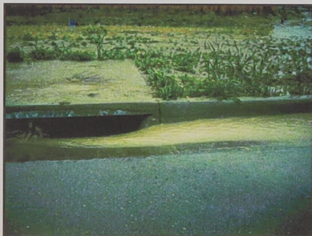
Figure 1.8 Sediment washed into a catch basin during a storm event.
