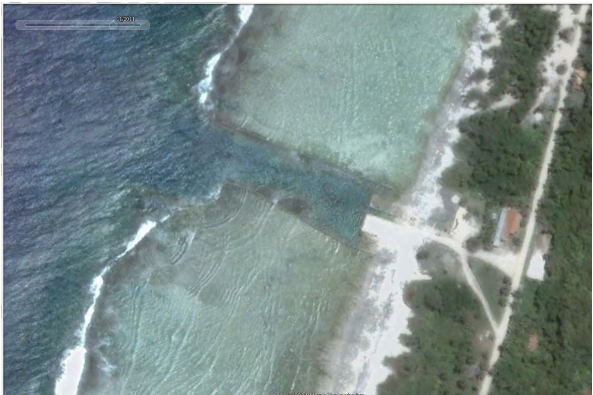
Figure 2.2-7: Mangaia harbour recorded 21 NOV 2011
