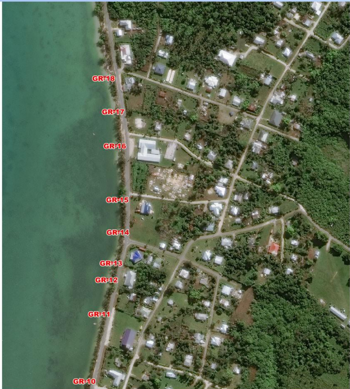
Figure 4.3.1-03: Display of groyne of image subset 02. Every groyne has a unique ID. The corresponding GIS layers allow a zoom in, see figures 4.3.1-01
