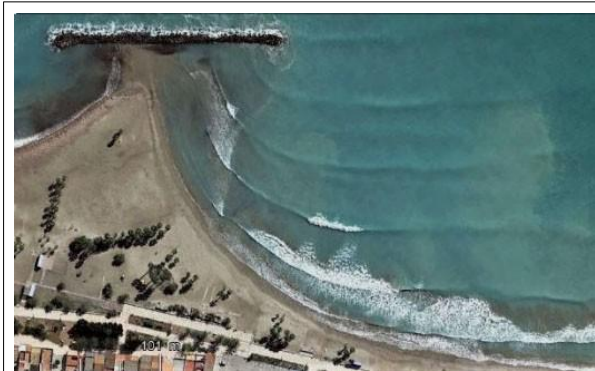
Figure 5.1-03: Detached breakwater (internet)
