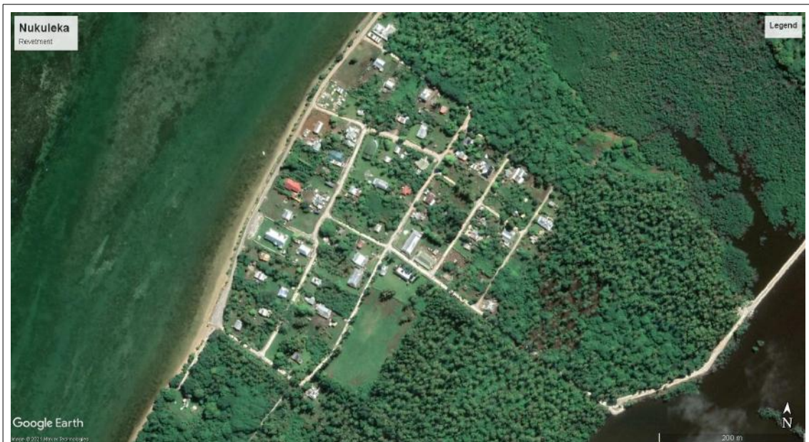
Figure 3.5-01: Nukuleka recorded July 2021. A revetment is currently not visible with very high resolution image data.
