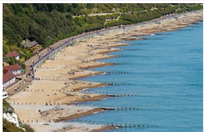
Figure 4.1-02: Beach groyne structures in Portugal
