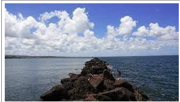
Figure 5.1-01: Breakwater at Suva Point during high tide
