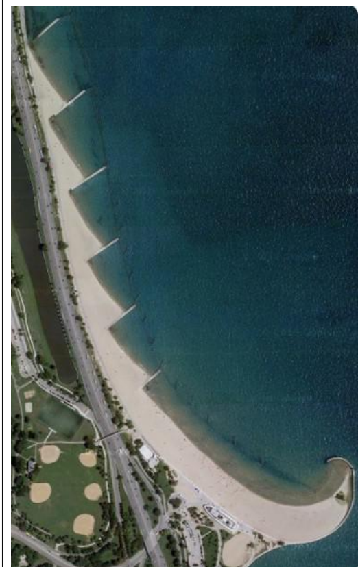
Figure 4.1-03: Satellite image of groyne structures with accumulated sand.
