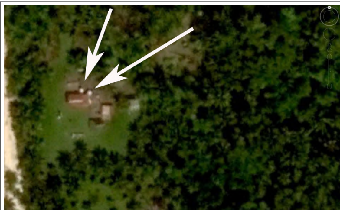
Figure 5.1.2-01: Zooming in allows to recognise infrastructure which could be concrete rain water tanks.
