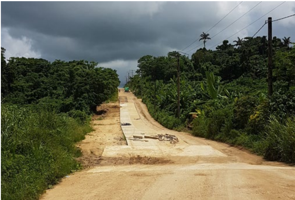
Plate 7 Legal road approach to landfill showing partly constructed concrete pavement on incline
