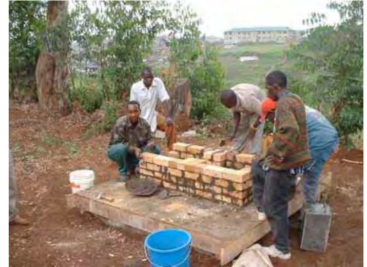
Photo 1: building the brick body
