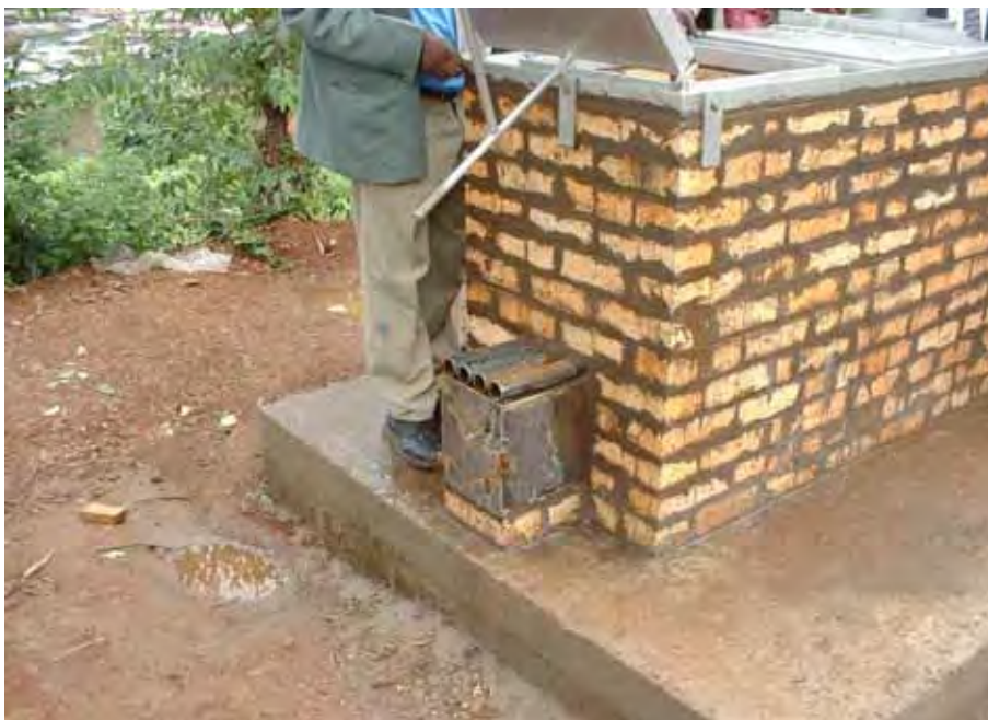
Photo 5: ash door, ash tunnel and air ducts
