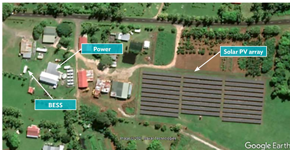
Figure 2.3: Example of Medium-Scale Project (Aitutaki, Cook Islands) (750 kW solar PV and 500 kW / 500 kWh BESS)
