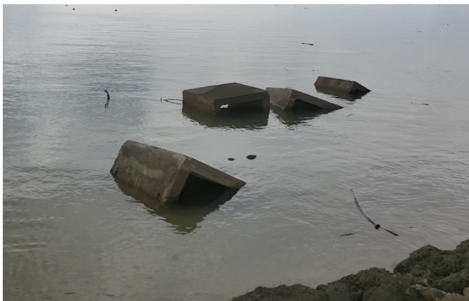
Figure 11. Groyne structure at Hahake completely disfigured by the recent Tsunami, 15th January 2022.
