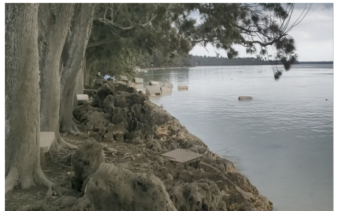
Figure 11. Groyne structure at Hahake completely disfigured by the recent Tsunami, 15th January 2022.
