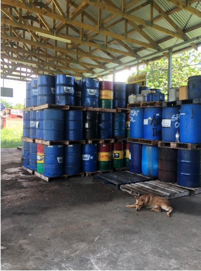
Figure 3. Storage inside of SWOMP facility. Visible black staining on flooring from spills.
