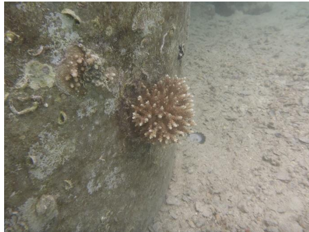
Encrusting coral on a wharf pile
