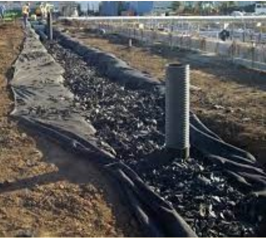
Figure 8: ELT replacing gravel in LFG extraction well
