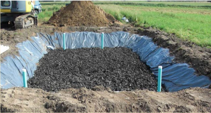
Figure 11: ELT used as drainage material in Septic Tanks
