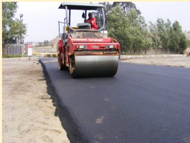
Figure 13: Rubber Crumbs used in Asphalt
