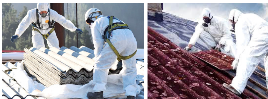
Removal of asbestos roofing. 11
