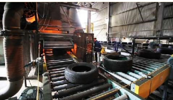
Figure 4: Injection of ELT into Kiln
