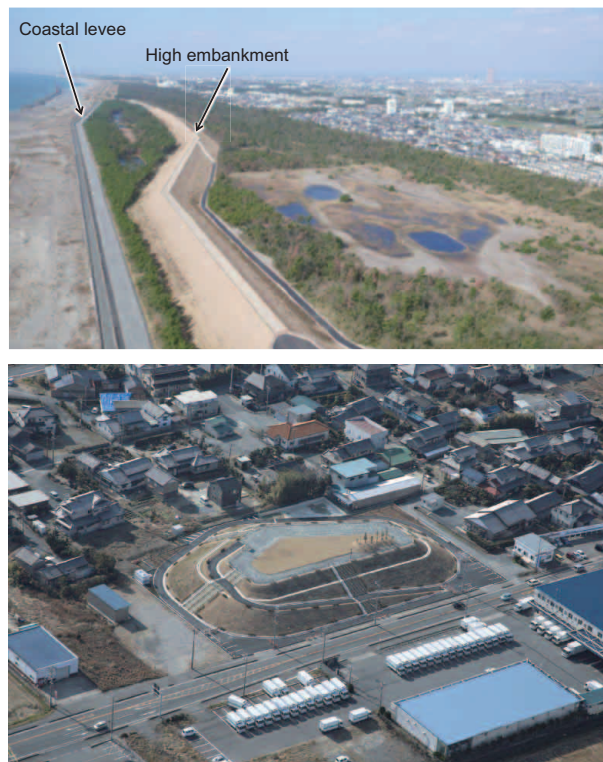
Figure 5-3-5 Top: High embankments built along the land side of coastal levees (Hamamatsu City) Bottom: “Life saver hill” (Fukuroi City) (provided by Shizuoka Prefecture)
