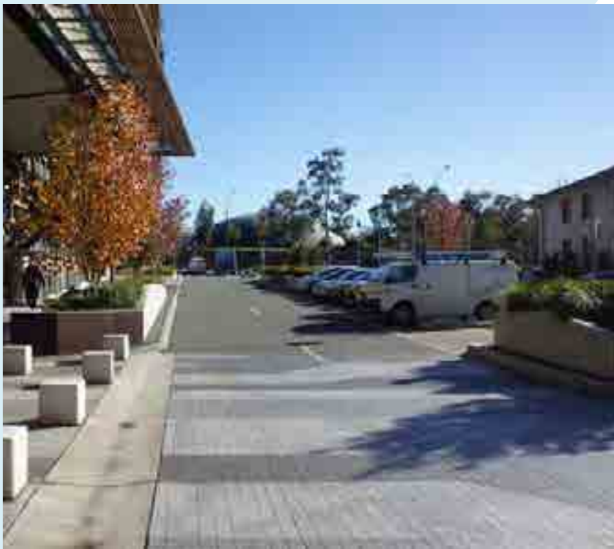
Figure 3.14: Example of raised road pavement in Canberra, Australia
