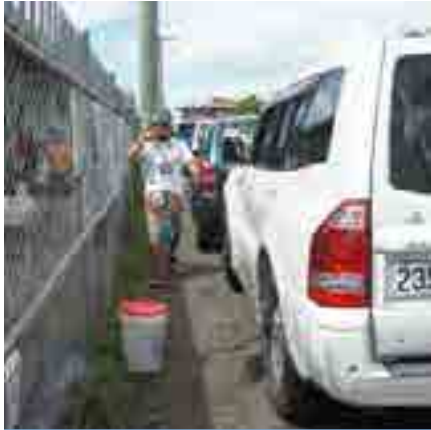
Existing infrastructure limits continuous access through the waterfront. Connectivity needs to be improved
