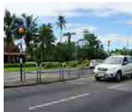
Figure 3.16: Pedestrian crossing with raised pavement, refuge and lighting
