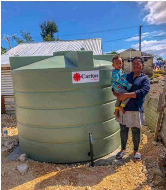
Fakei Latu and her baby next to a water tank installed outside her house. The tank serves 19 people around low lying Pa Tangata near Nuku'alofa, Tonga.
