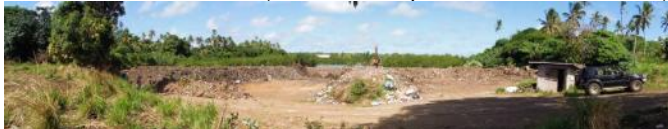
(2. Karaka dump site, during rehabilitation)
