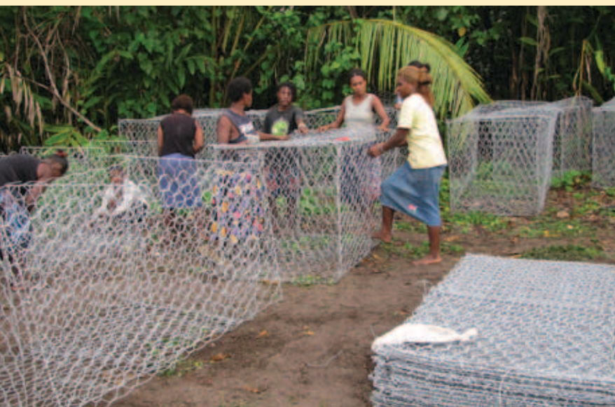
Women making gabion baskets. Makira, Solomon Islands
