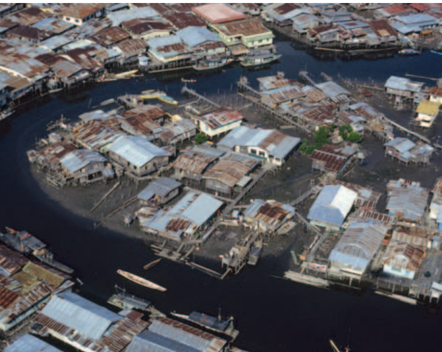
Growth of informal settlements contributing to increasing vulnerability is a typical feature of many Asian cities. Sandakan City, Malaysia
