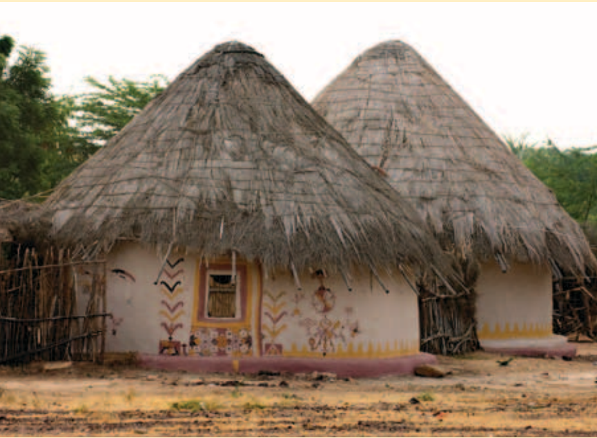
Traditional circular construction of huts is safer in seismic areas, Gujarat, India'
