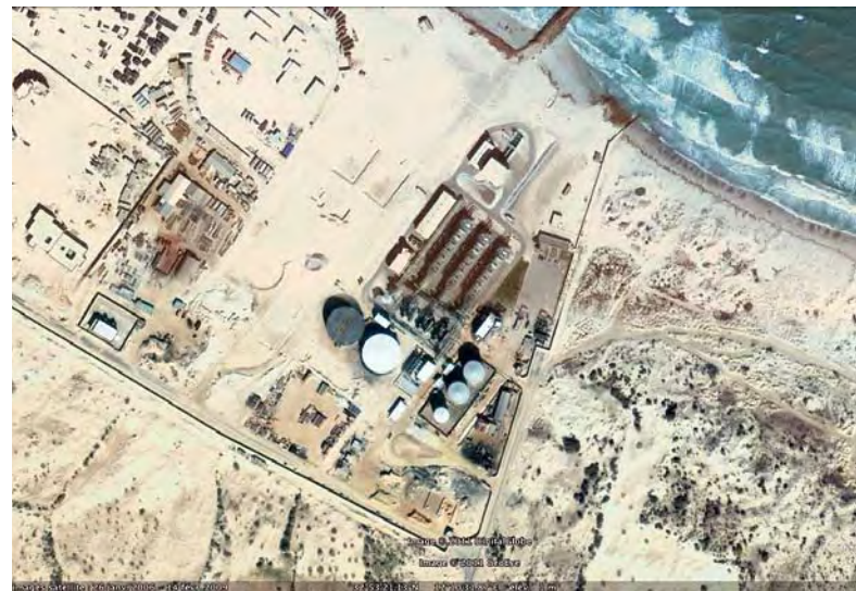
Zuwarah desalination plant (Nalut). © GoogleEarth.
