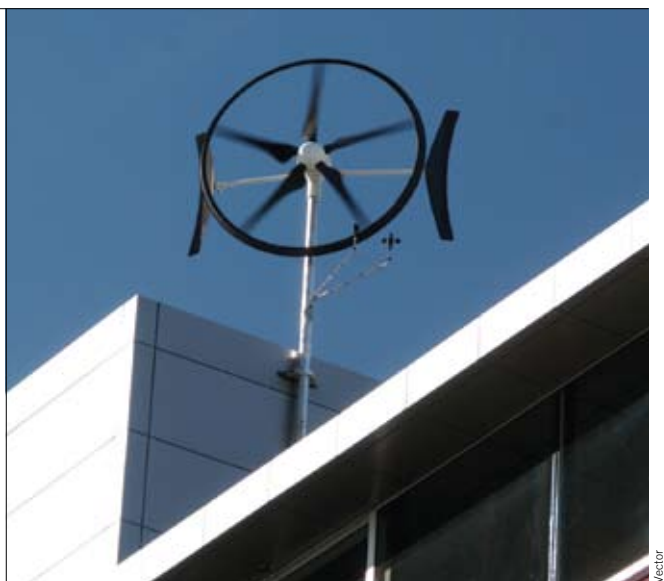
This Swift Turbine is mounted on the Waitakere City Council building at Henderson, Auckland, for a trial by Vector. The turbine is about 2 metres in diameter and weighs about 50 kilograms. It could provide about a quarter of an average New Zealand household's annual electricity use.
