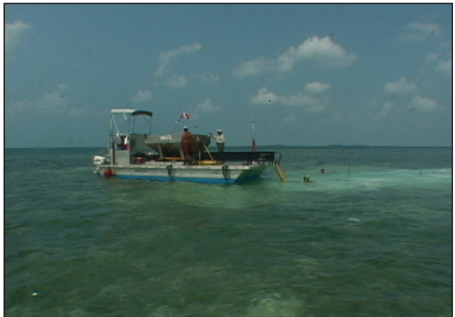
Figure 18.4. Restoration of seagrass beds damaged by a vessel grounding required the addition of gravel substrate at Calda Bank off Key West, Florida. Photo: A. Farner.
