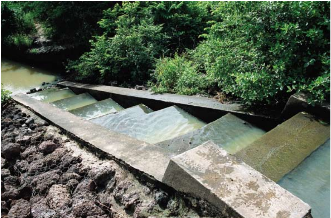
Photo 3.2 Fish ladder enables fish to migrate beyond irrigation dam (Burkina Faso). Fish ladders are an important infrastructure improvement that can accompany environmental flow releases.
