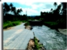
Erosion causing road loss in Vanuatu
