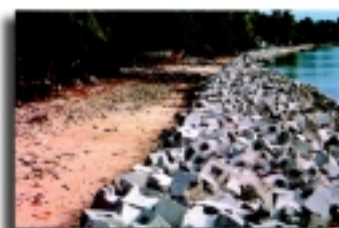
Concrete bricks acting as coastal protection structures
