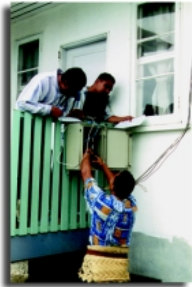
Installation of photovoltaic cells
