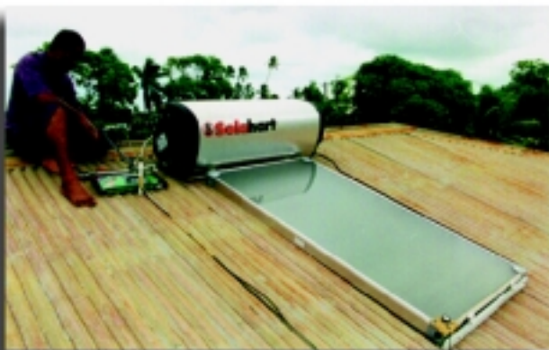
Installation of solar photovoltaic cell
