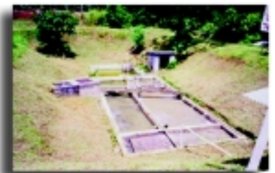
Sewage plant in Tonga
