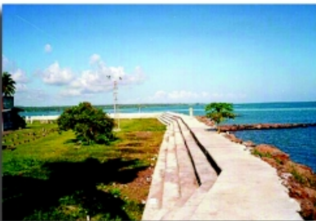
Coastal protection structure in Apia
