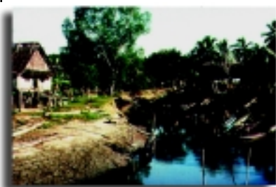
Water-front houses in PNG - erosion threats are high
