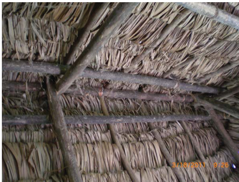
Figure 10. The ridgepole ( saqai ) that supports the thatched roof.
