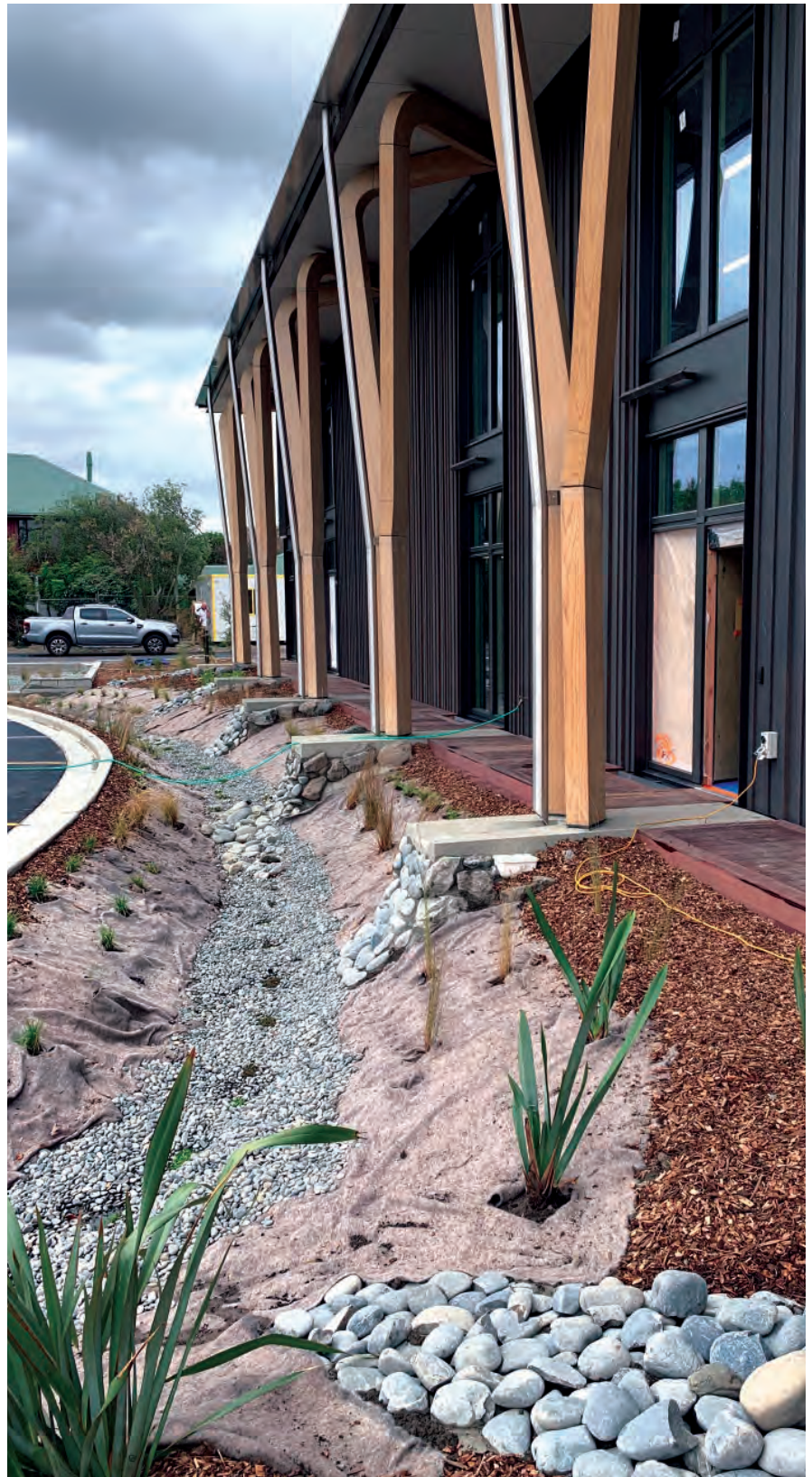
Rainwater from the office wing of our Te Rauhitanga building is channelled into a rain garden. We will harvest water from the main office roof for use in the building.
