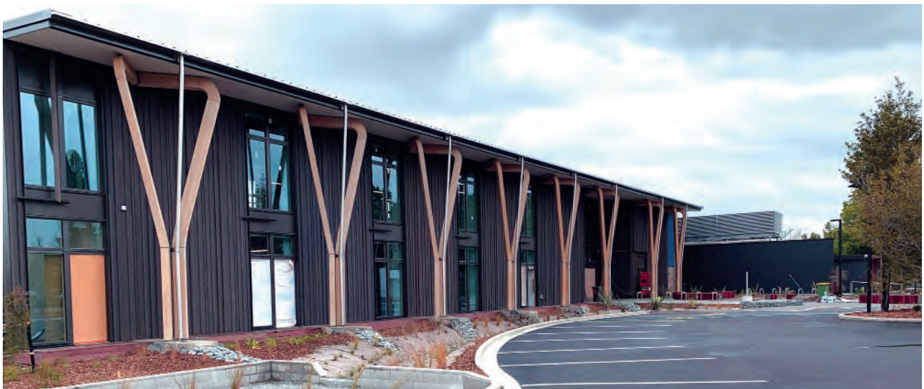
A view of the new Lincoln office; Te Rauhitanga – the gathering place.
