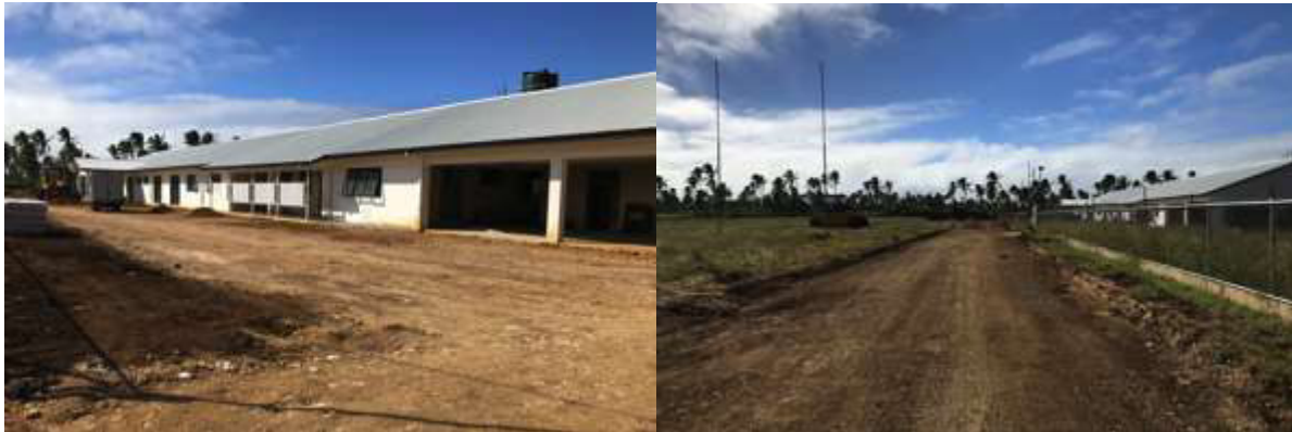
Figure 12 Ha'apai Hospital Front View (Left), Access Rd. (Right)
