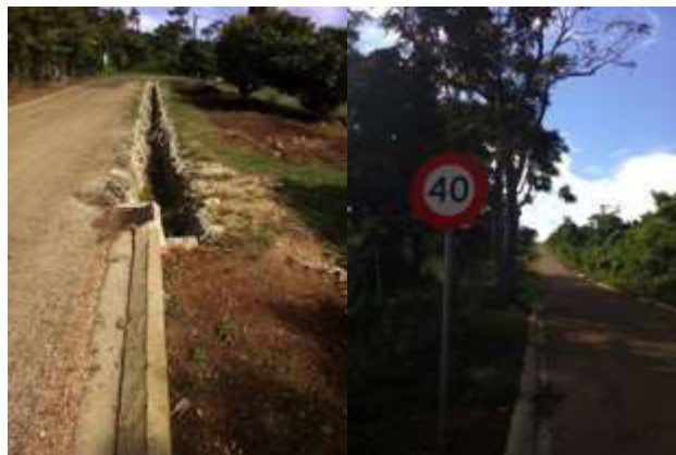
Figure 15: Tufuvai Evac. Road. Road Furniture's Q2 2019 (right).
