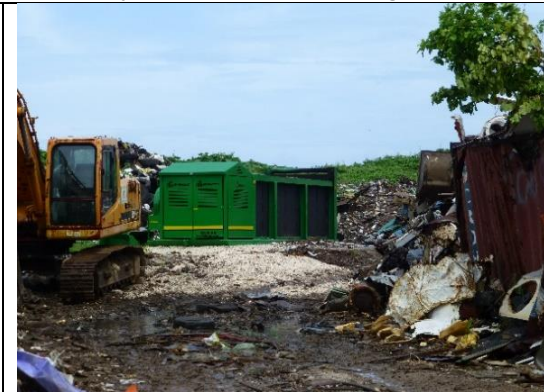
The incinerator was installed at the final disposal site to reduce incoming waste for land-filling. (Operation has ceased as of May 2019.)
