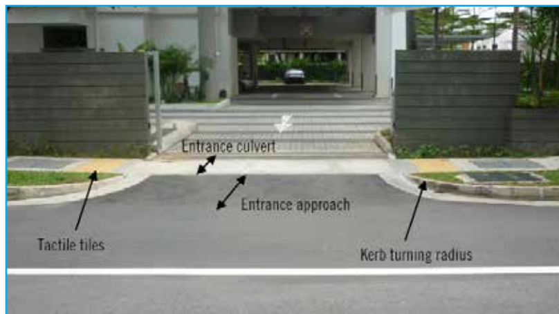
Accessibility Features at Driveway Entrance
