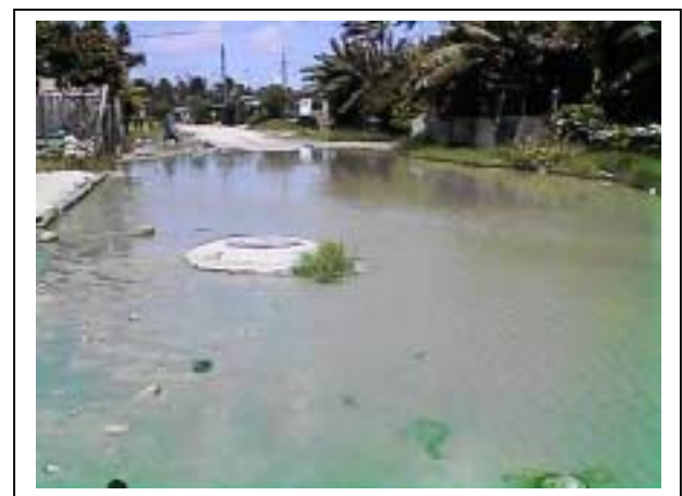
Figure 6. Poor Drainage in Majuro
