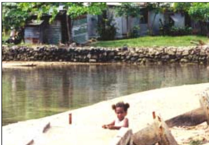
Figure 4.6. A Seawall in Qoma, Fiji
