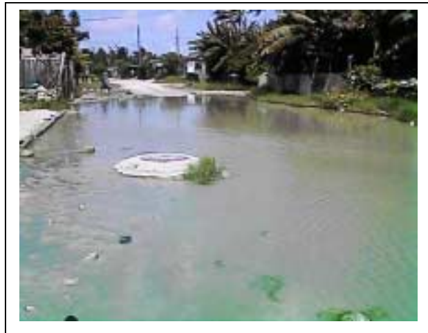
Figure 2.3. Poor Drainage in Majuro
