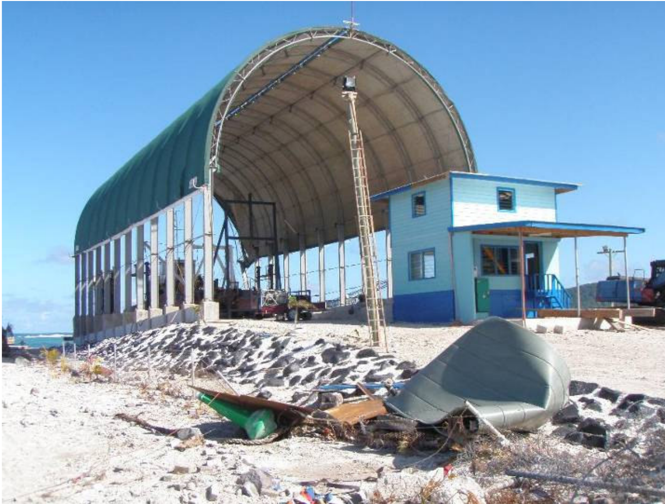
Plate 2: Damaged wharf, Satitua (High impact)
