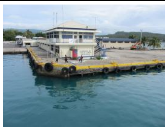
Figure 4-46 Entire view of Salelologa Port
