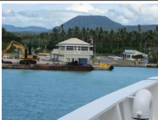
Figure 4-45 Entire view of Mulifanua Port
