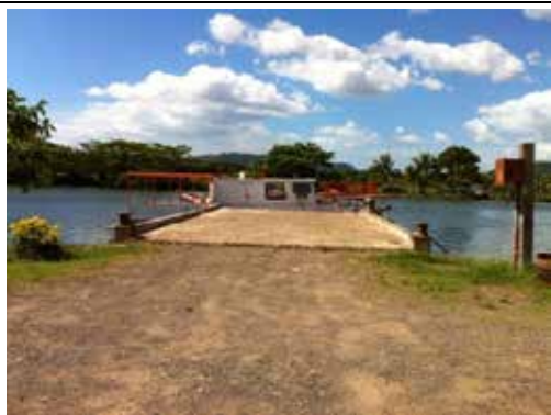
Figure 4-30 Entire view of Labasa Jetty
