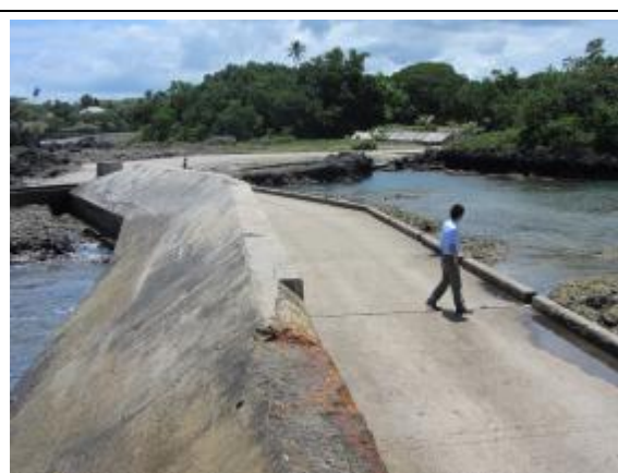
Figure 4-63 Approach road to Lenakel Wharf
