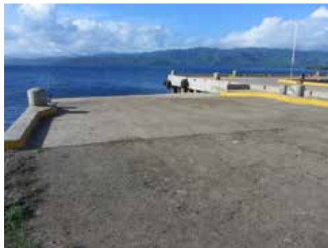
Figure 4-28 Ramp of SavuSavu Jetty to which Ro-Ro boats are moored (longitudinal mooring)
