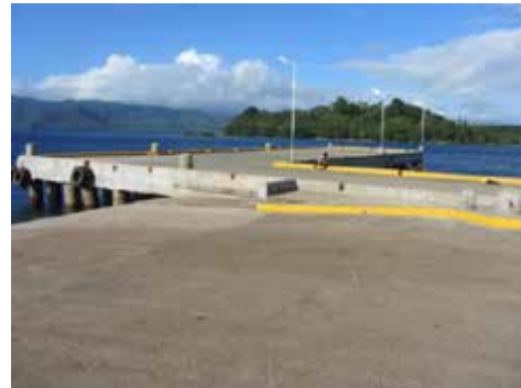
Figure 4-29 Newly constructed mooring jetty at SavuSavu Jetty
