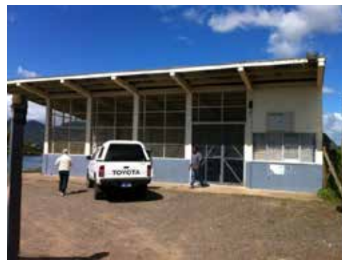
Figure 4-31 Office building of MSAF
