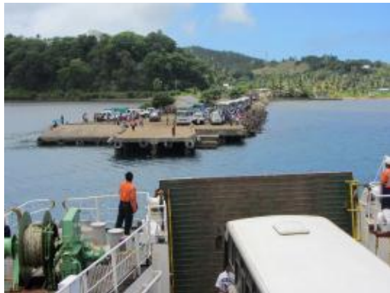
Figure 4-26 Entire view of Nabouwalu Jetty
