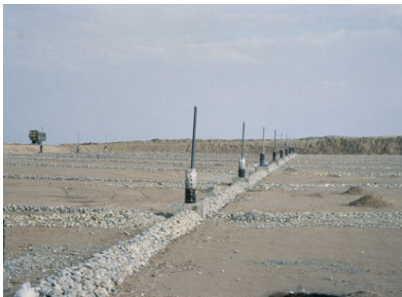
Picture 2-15 Installation example of gas venting pipes
