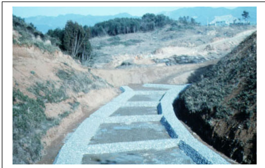
Picture 2-9 Placement example of leachate collection discharge pipes at Fukuoka-shi Busetsugaura Landfill
