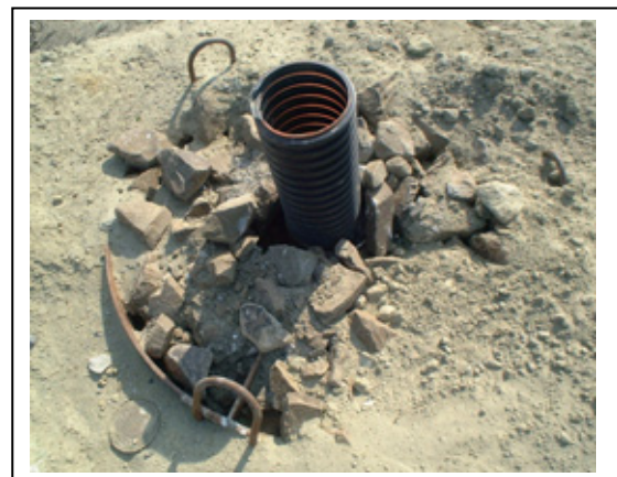
Picture 3-5 Gas venting facility that is in the process of being plugged and buried (bad example)
