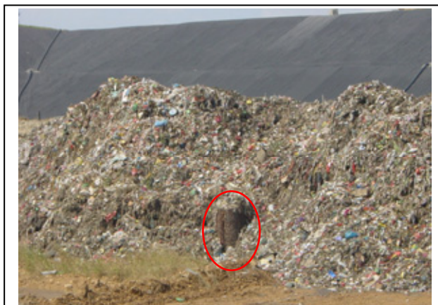
Picture 3-4 Waste is higher than Gas venting facility (○) case (bad example)
