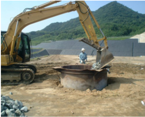
Picture 3-7, 8 Construction example of raising post construction type gas venting facilities
