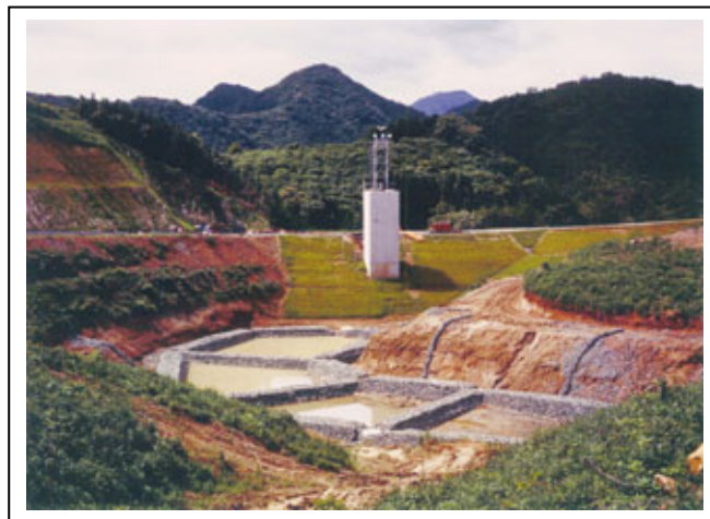
Picture 2-8 Example of pit pump method
