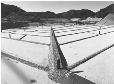
Picture2-11 Good example of leachate collection facilities
