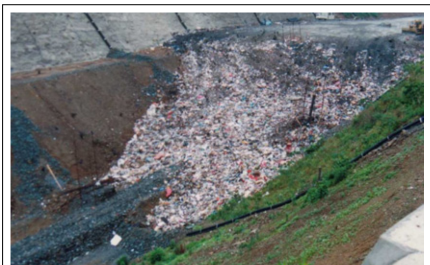
Picture 3-2 Example of landfill of large waste material in the vicinity of leachate collection discharge pipes
