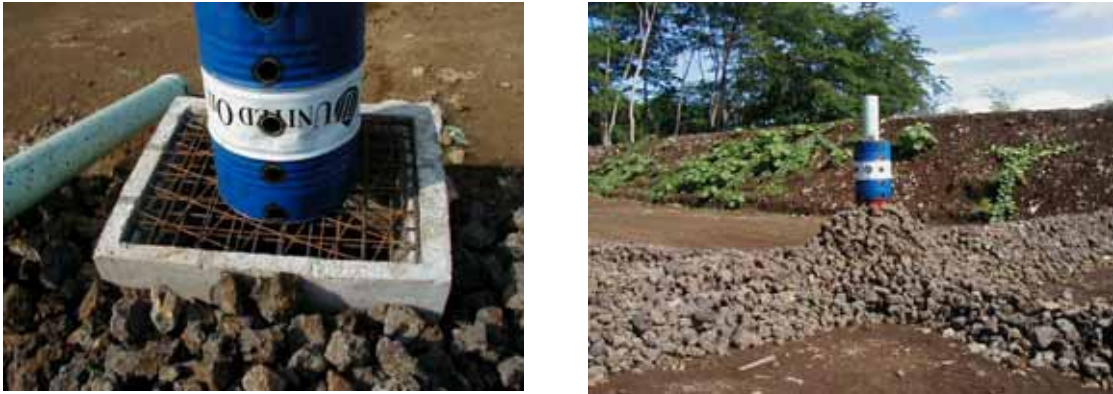
Photo- 23: Vertical Gas Venting Pipe installed on Pipe Connection Pit
