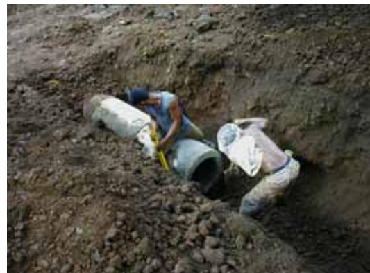
Photo- 12: Diversion Pipe Setting
