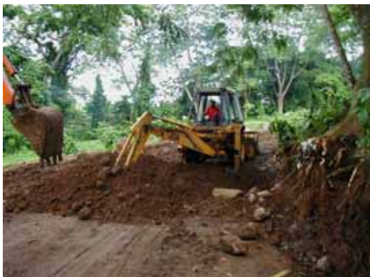
Photo- 11: Excavation of Trench
