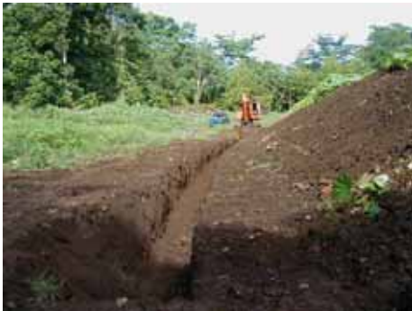
Photo- 10: Perimeter Drain Excavation
