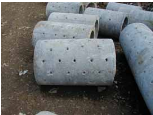
Photo- 14: Leachate Collection Pipe
