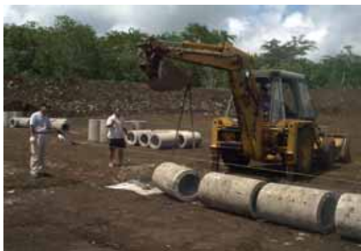
Photo- 16: Concrete Pipe Setting
