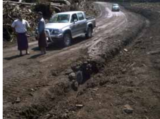
Photo- 9: Side Ditch with Road Crossing Culvert
