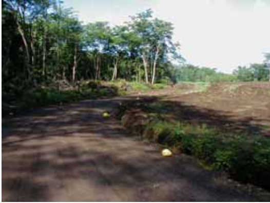
Photo- 8: Side Ditch with Curb Stone
