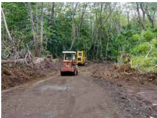
Photo- 6: Compaction & Gravel Paving
