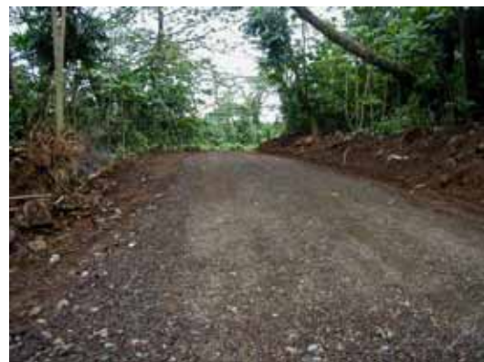
Photo- 7: Paved Access Road
