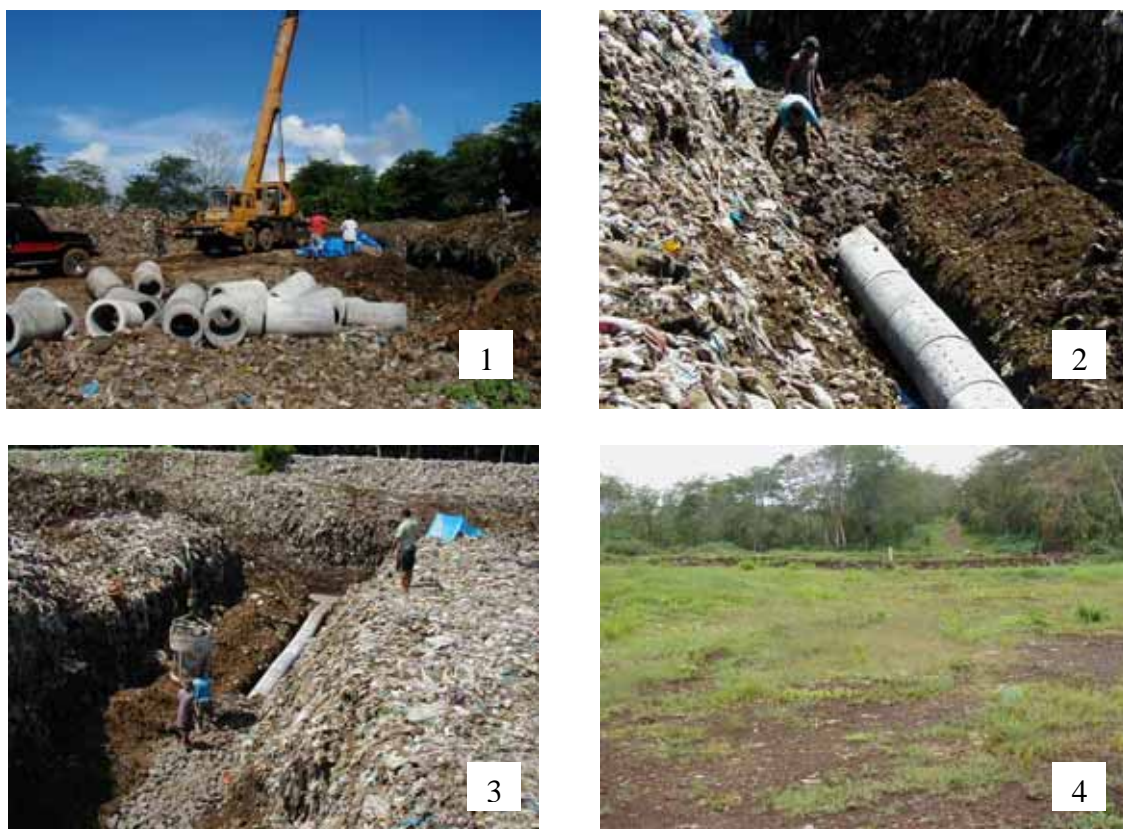
Photo- 19: Installation of Leachate Collection Facility at Deep Waste Layer
