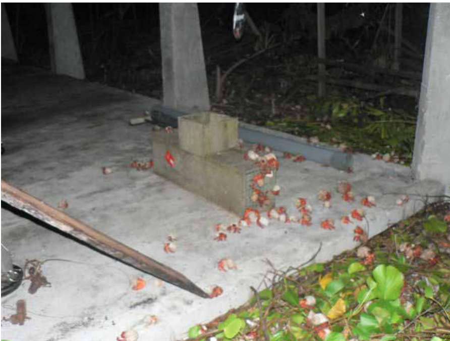
FIGURE 6.9 – Chimney box and ramp showing crab exclusion.
